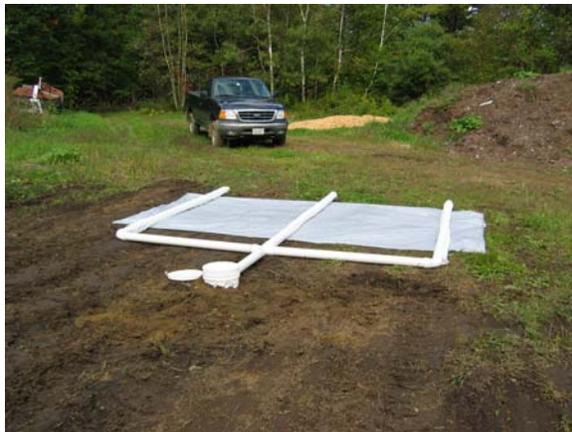
Figure 2. Photograph depicting “Leachate Collection System”, prior to construction of Pile #3.
